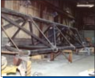
Reduced Premature Cracking. U.S. Navy.
